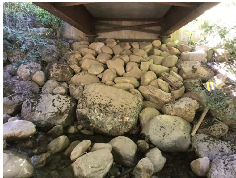
Left Bank Abutment when facing downstream
