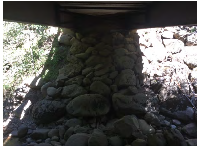
Right Bank Abutment when facing downstream
